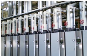
Asahi Soft Drinks Co., Ltd. Fuel conversion Once-through boiler: 2.5 t/h × 15 Once-through boiler: 1 t/h × 1 (relocated)
