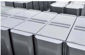
Osaka Prefecture Bloom Energy Japan Ltd. Fuel cell batteries Generation capacity: 1,200 kW (200 kW × 6 systems)
