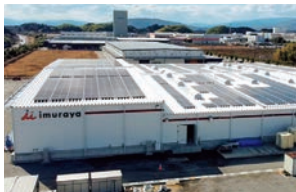
IMURAYA GROUP CO., LTD. (Anotsu FACTORY) Generation capacity: 668.16kW (Hanwha Q cells 580W × 1,152 panels) Module type: monocrystalline *On-site PPA(Combined with battery storage) Large battery storage Capacity: 1,000 kWh class(Huawei output, 300kW)
