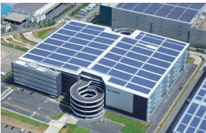
GLP Japan Inc. (GLP Zama Solar Power Plant) Generation capacity: 2,250.50 kW (Yingli Solar 250 W × 9,002 panels) Module type: polycrystalline
