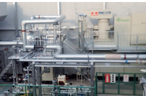
Tsurumi Paper Co., Ltd. Cogeneration system Generation capacity: 1,660 kW Steam output: 5,150 kg/h
