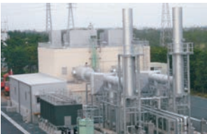
Kashima Doryoku K.K. Cogeneration system Generation capacity: 5,750 kW × 2 units Flue gas steam boilers: 2.9 t/h × 2 units
