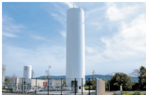
Meiji Co., Ltd. LNG satellite facility Storage capacity: 100 kL Steam-heated vaporizer: 400 kg/h × 1 Low-temperature water-heated vaporizer: 500 kg/h × 1
