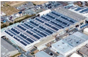
THK Rhythm Co., Ltd. Generation capacity: 1,829.52 kW (Trina Solar 495 W × 3,696 panels) Module type: monocrystalline *On-site PPA
